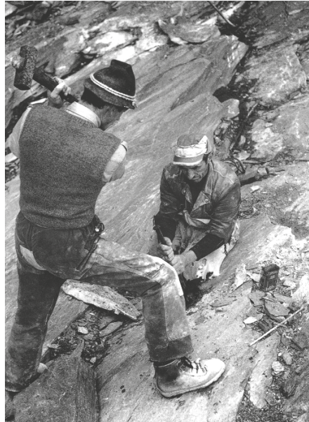
Manual preparation of the borehole for an explosive charge.
